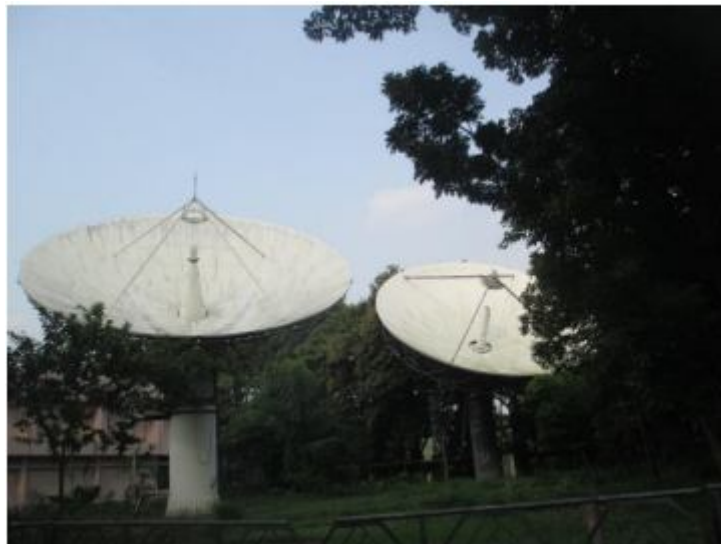
Fig 6.2: Mohakhali Earth Station
